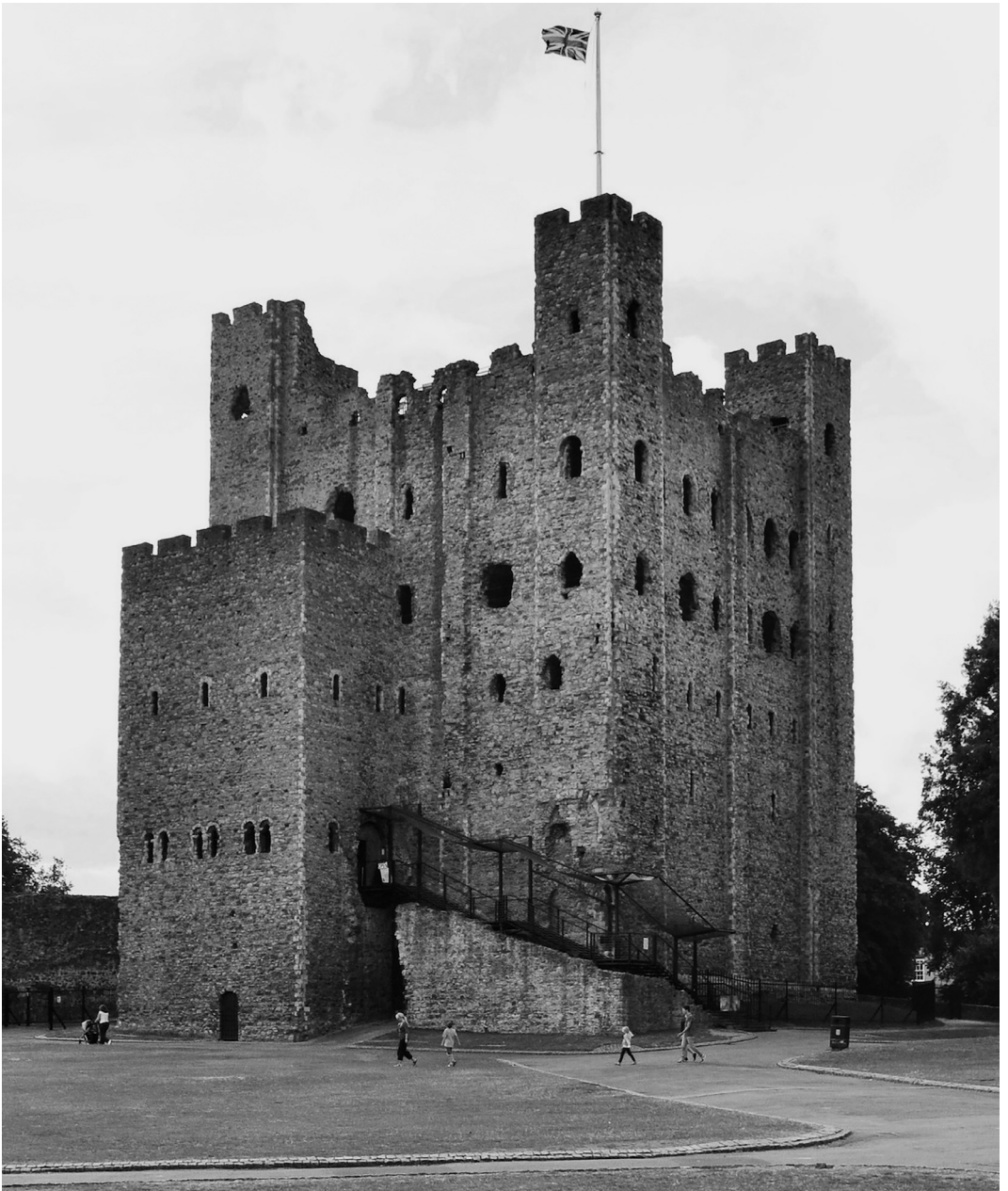
Rochester: The great tower (c.1130) from the NE.
